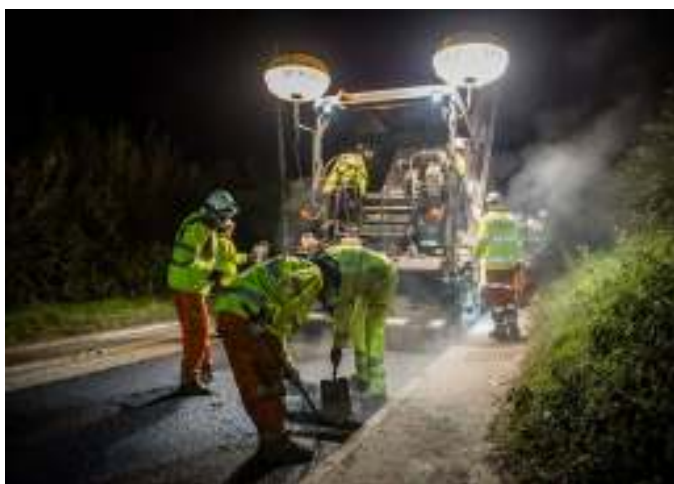
Figure 11: Highway Maintenance xiv
